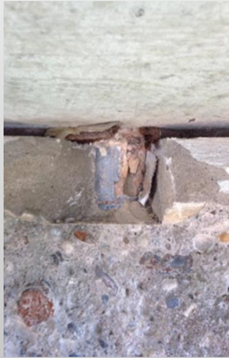
Bridge 2 Spalling
